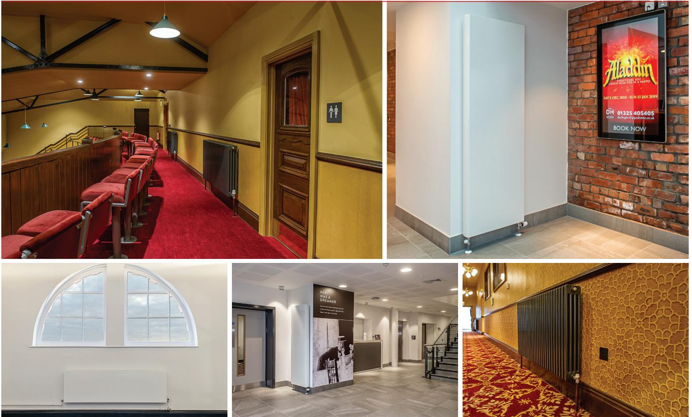
The building is heated using a gas fired condensing boiler and heat is managed in zones to make the most efficient use of energy. Each zone has been fitted with a selection of different Myson radiators which blend with the style while effectively delivering a comfortable warmth both front and rear of house.
